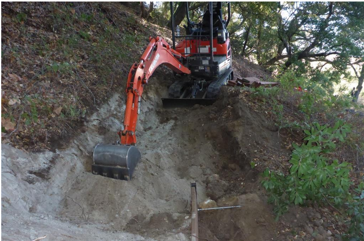
Narrow footprint excavator for excavation work on and near trails. Photo credit: Adam Maywhort.
