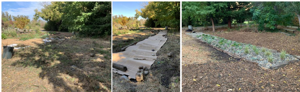
Sheet mulching sequence to create a bioswale. Photo credits: Kimberly Crispin.
